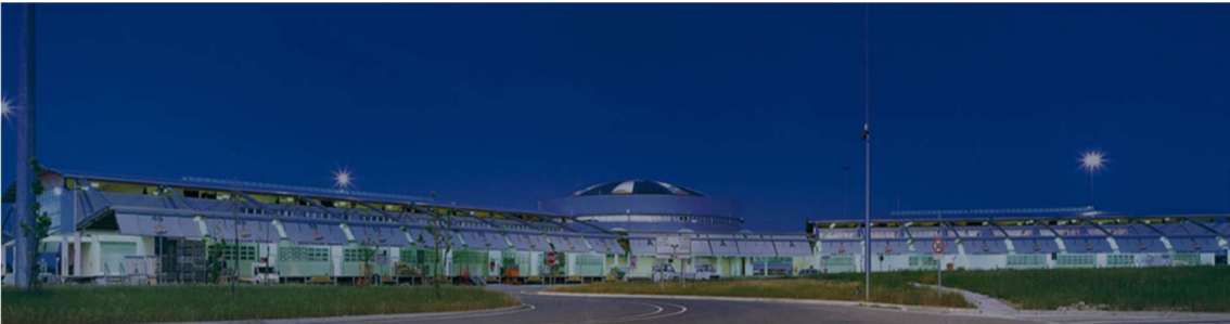
Figure 8 : External view of the complex
