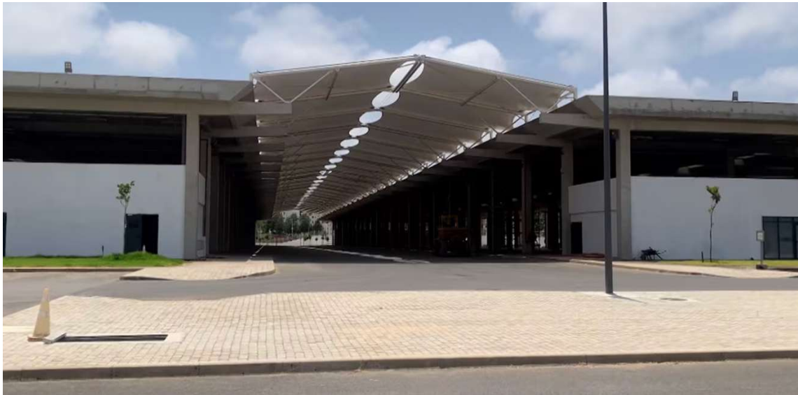
Figure 11 : External view of the market
