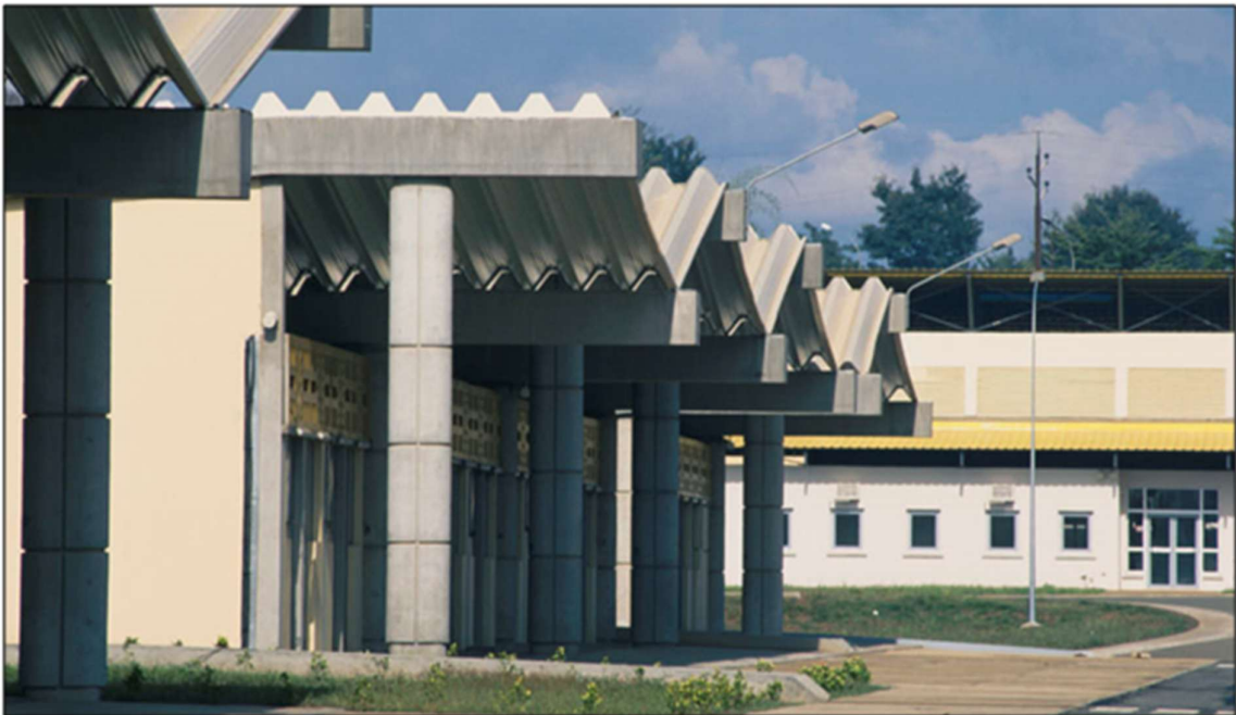
Figure 17 : External view of the market
