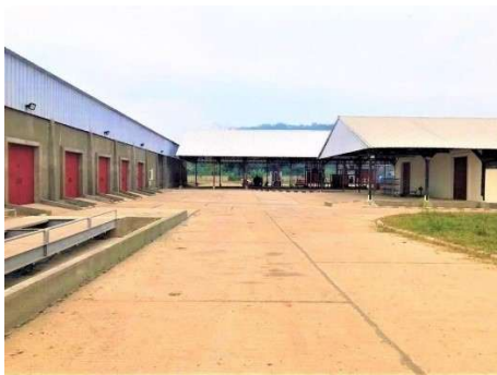
Figure 2 : Buildings of the complex
