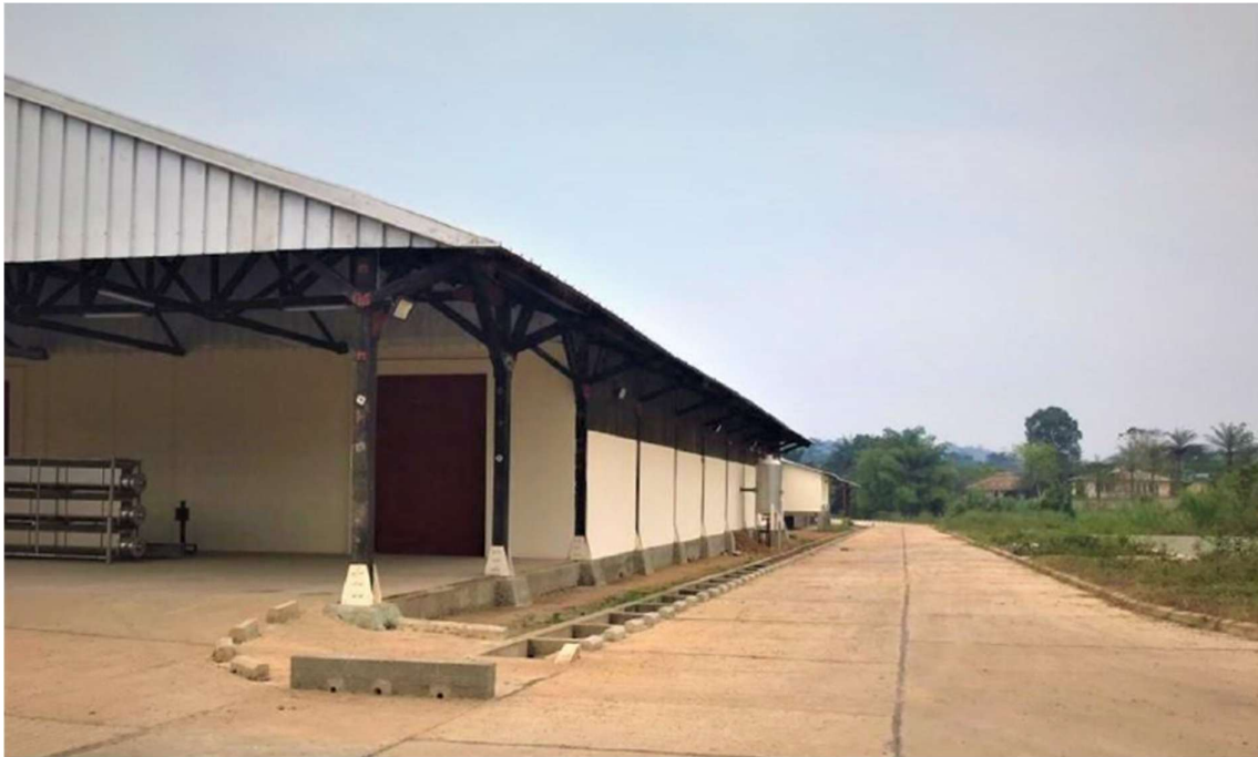
Figure 4 : External view of a building in the complex
